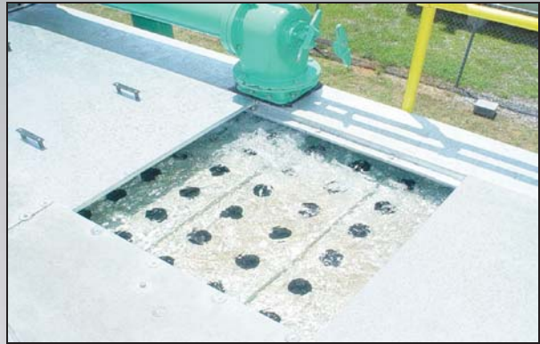
EVAPCO Hot Water Basin Replacement
