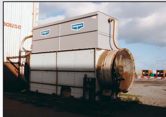
EVAPCO Coil Casing Replacement
